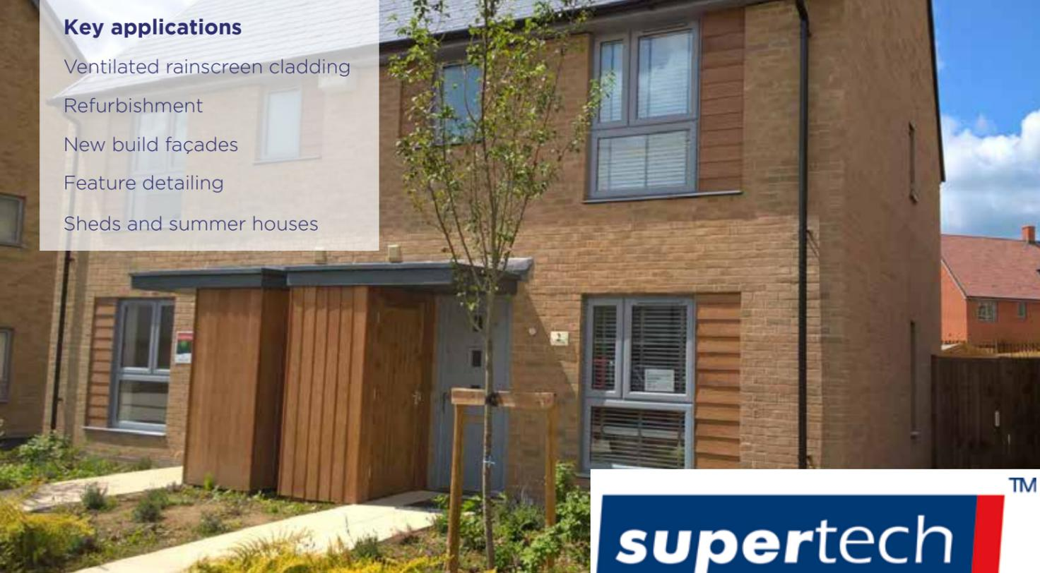
Supertech Weatherboard is a simple to install, fully ventilated rainscreen cladding system which has an appearance similar to that of timber but the durability and strength of cement.
